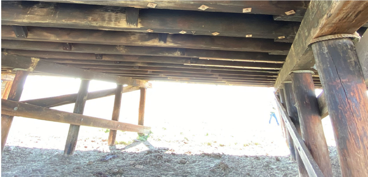
Picture 3 – Existing beam lag bolts
