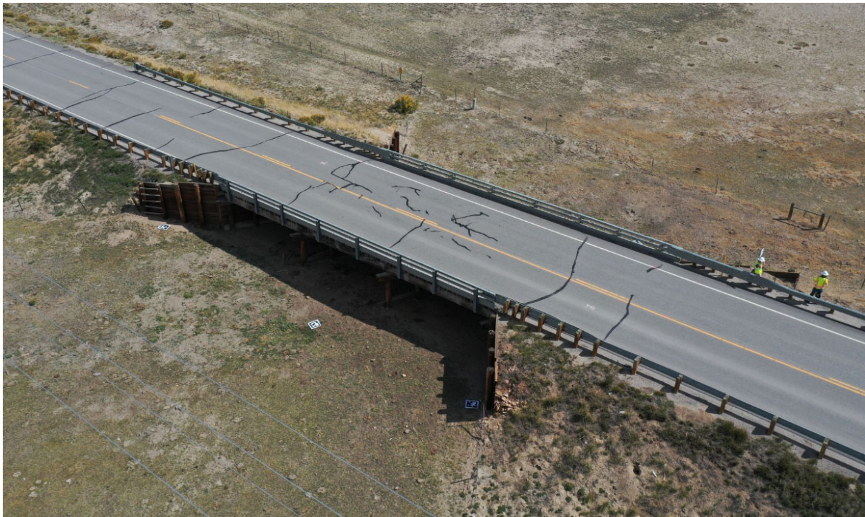
Picture 1 – Bridge I-13-H General Location
